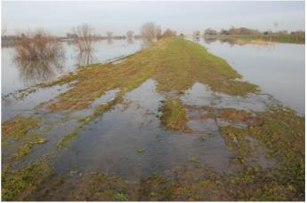
When the water level in the reservoir reaches the Cradge Bank's crest it is storing approximately 90,000,000 cubic metres of water above the surrounding ground. This is enough water to fill Wembley Stadium 22 times.
